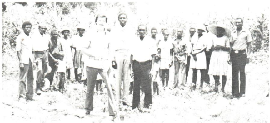
Breaking ground for Church School in Haiti.
